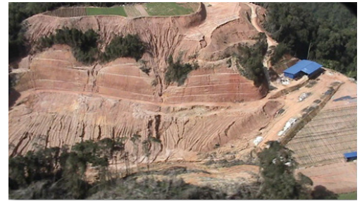
Illegal land clearance at Terla Post
