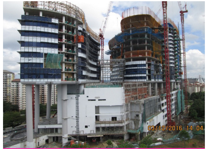
Construction of the new MACC Headquarters at Precinct 7, Putrajaya
