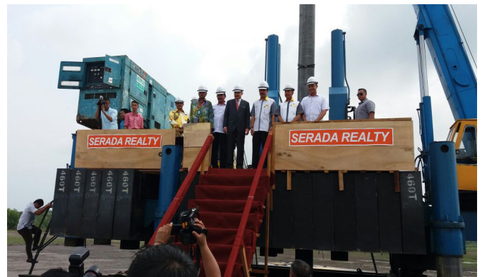
The ground-breaking event and works at the site of Terengganu MACC Office
